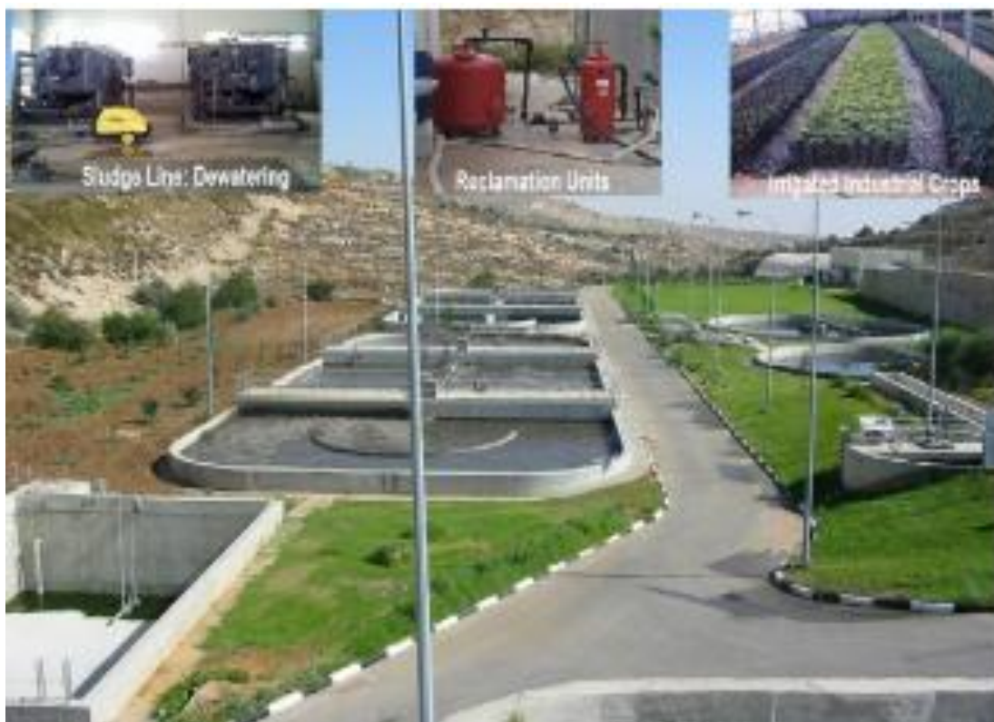
Fig 2.1 the different sectors of Al- Bireh treatment plant
